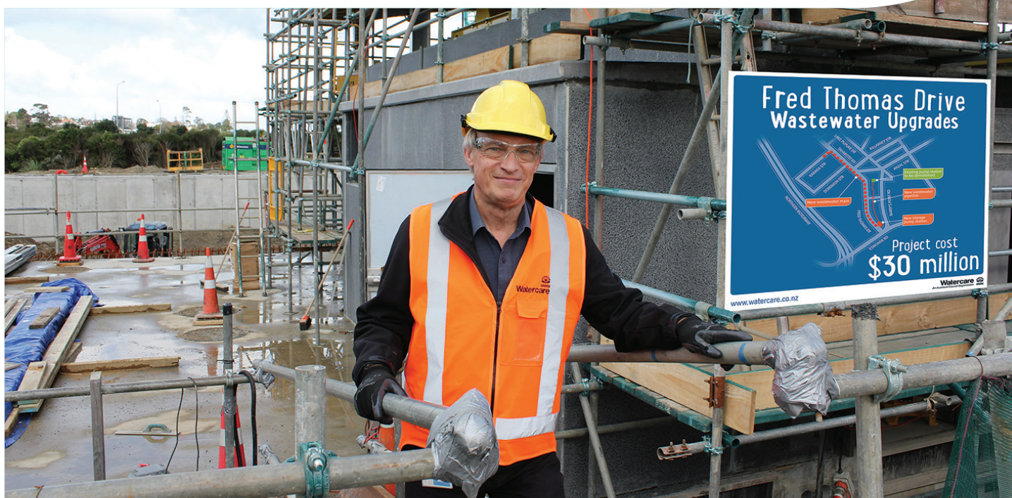
Project manager Ken Lukar at the site of the new pump station on Fred Thomas Drive.
